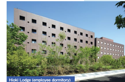
Hioki Lodge (employee dormitory)
