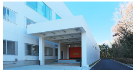
New truck terminal at head office factory
