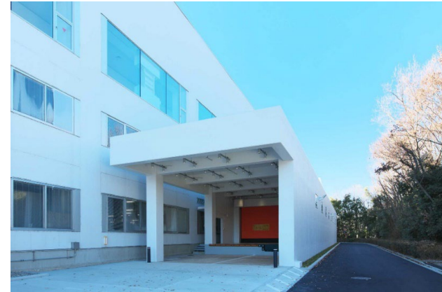
New truck terminal at the Head Office Plant
