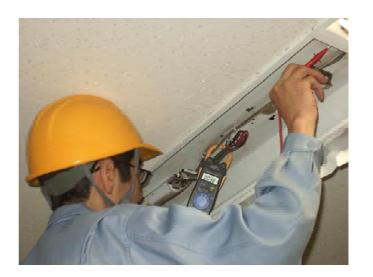
Note: The sensor part of the Clamp on HiTester is designed to be able to support the weight of the tester, but be careful not to apply excessive force to the sensor part and test lead wires by, for example, pulling the main body or test lead wires while the tester is clamped.
