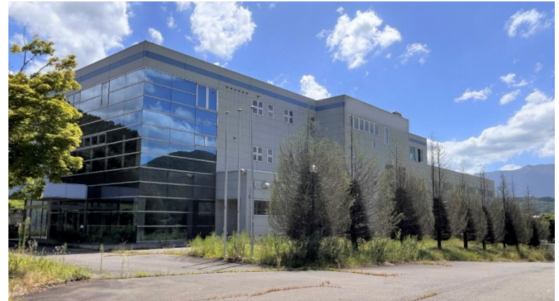
Ueda No. 2 Plant
